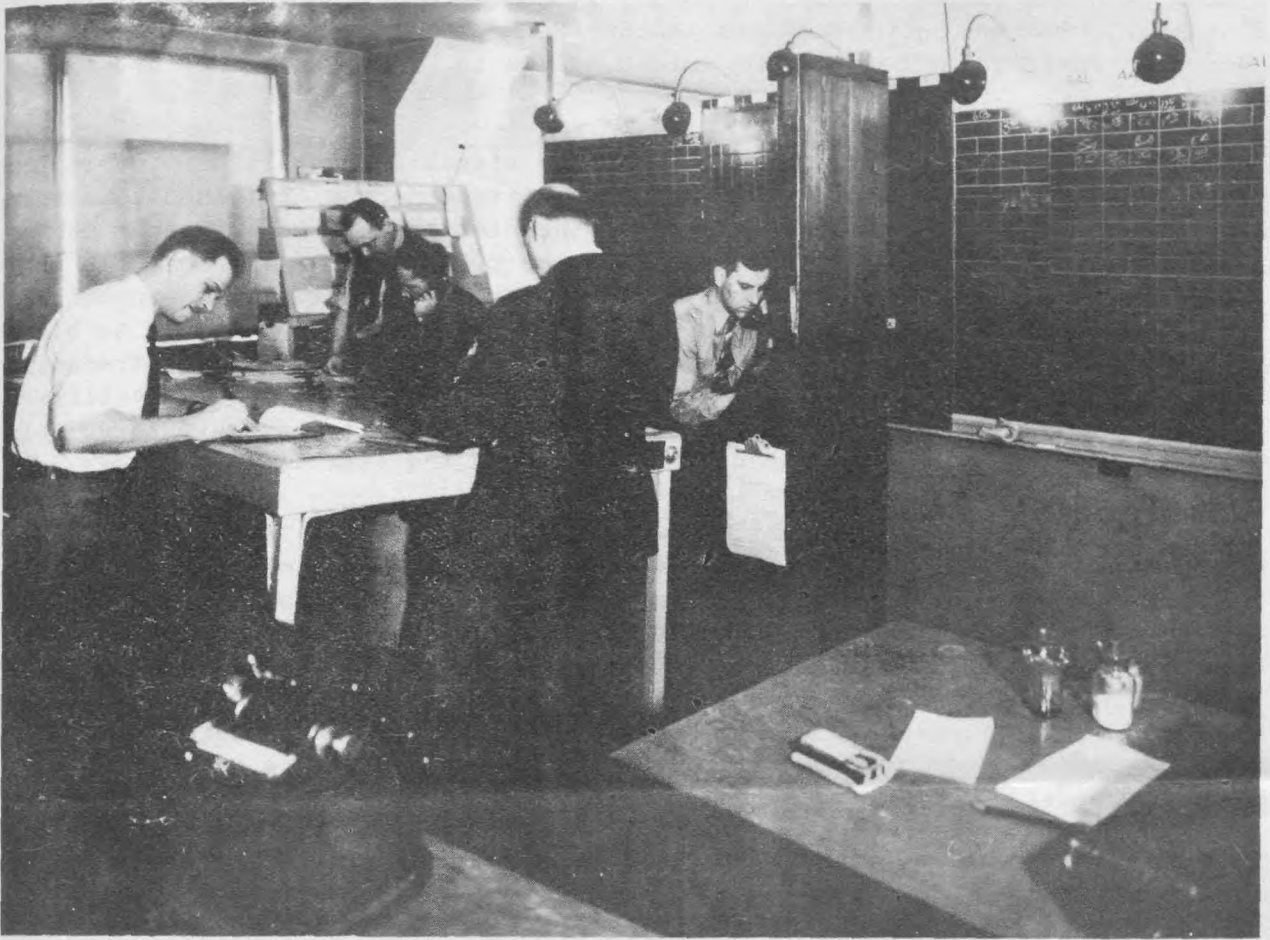
A section of the Airways Traffic Control office
