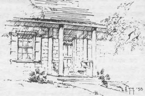
~ THE EAVES BECOME A STOOP ~ Drinkerhoff House
