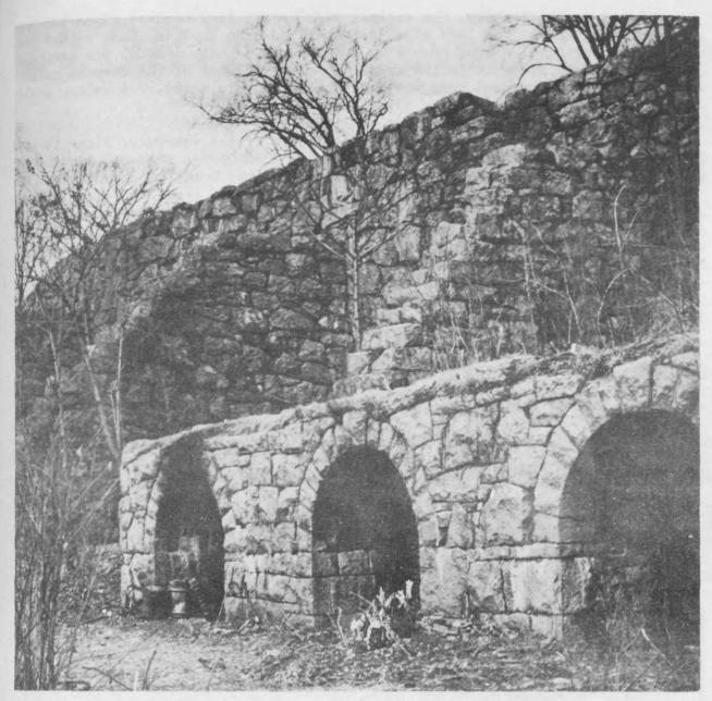
Huge stone walls, like this one at Boonton, were erected to keep the canal from washing away its banks and running over the lowlands. Some of the stones in this wall are almost ten feet long. No concrete was used in the construction—the stones are cut and fitted so perfectly that after years of service the wall is still in perfect condition.
