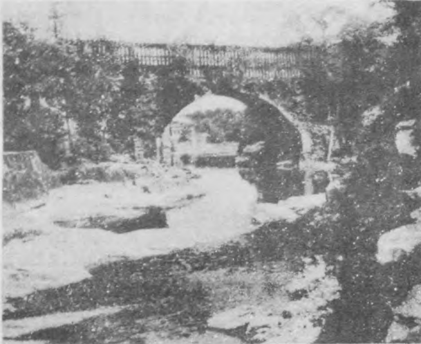
The Canal Crosses the Passaic River on an Aqueduct
