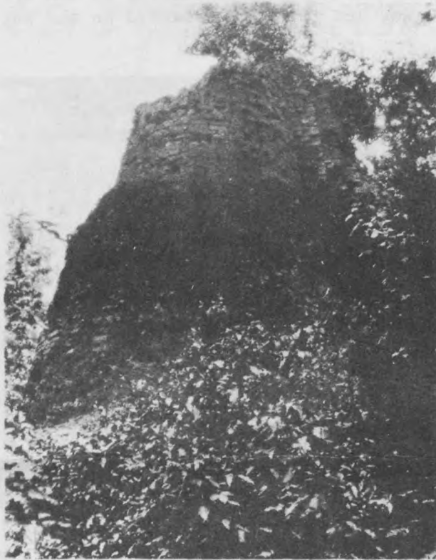
RUINS OF ETNA FURNACE SHOWING EXTERIOR AND VARIOUS LAYERS OF BRICK COMPOSING THE STACK
