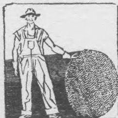
The George Washington Bridge Cable
