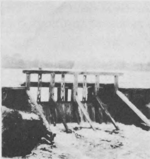
Flooding a bog
