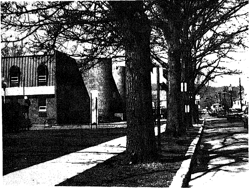
"Scotch Plains Municipal Building, Park Avenue"
