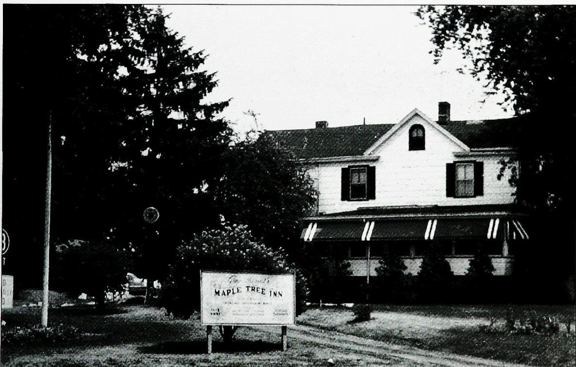
THE MAPLE TREE INN. Throughout the 1940s, 1950s, and 1960s, this inn, owned by Gene Laurent, with its sloping lawn and tree-filled grounds, was a popular dining and political gathering place. The inn faced onto South Avenue at the corner of Terrill Road, on the site now occupied by the Exxon service center.
