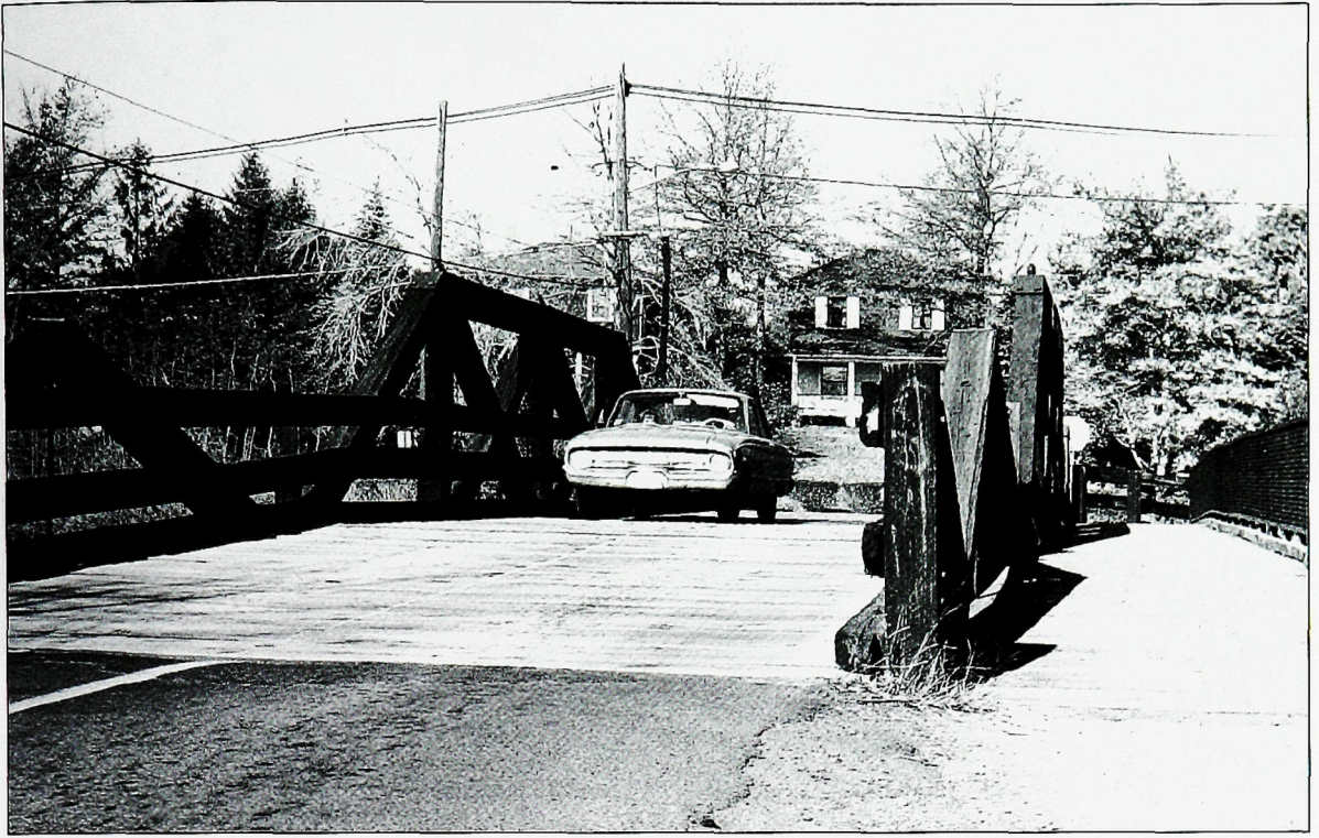
AN OLD PATHWAY. The wooden truss bridge at Sheelen's Crossing permitted passage over the railroad from North and South Avenues. By 1966, it had been replaced by a modern concrete structure.
