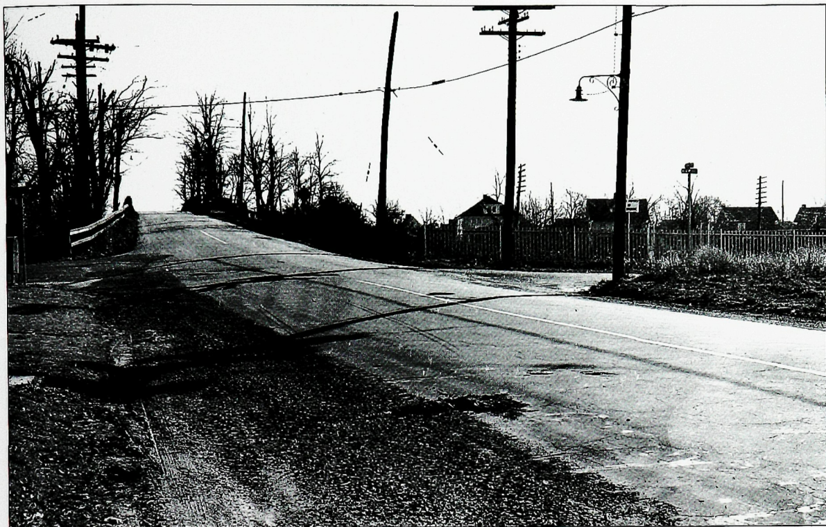
AN EARLY ROADWAY. This southward view on Terrill Road, a passageway that dates back to the Revolutionary War period, shows the narrow bridge over the railroad. North Avenue crosses over from left to the right.
