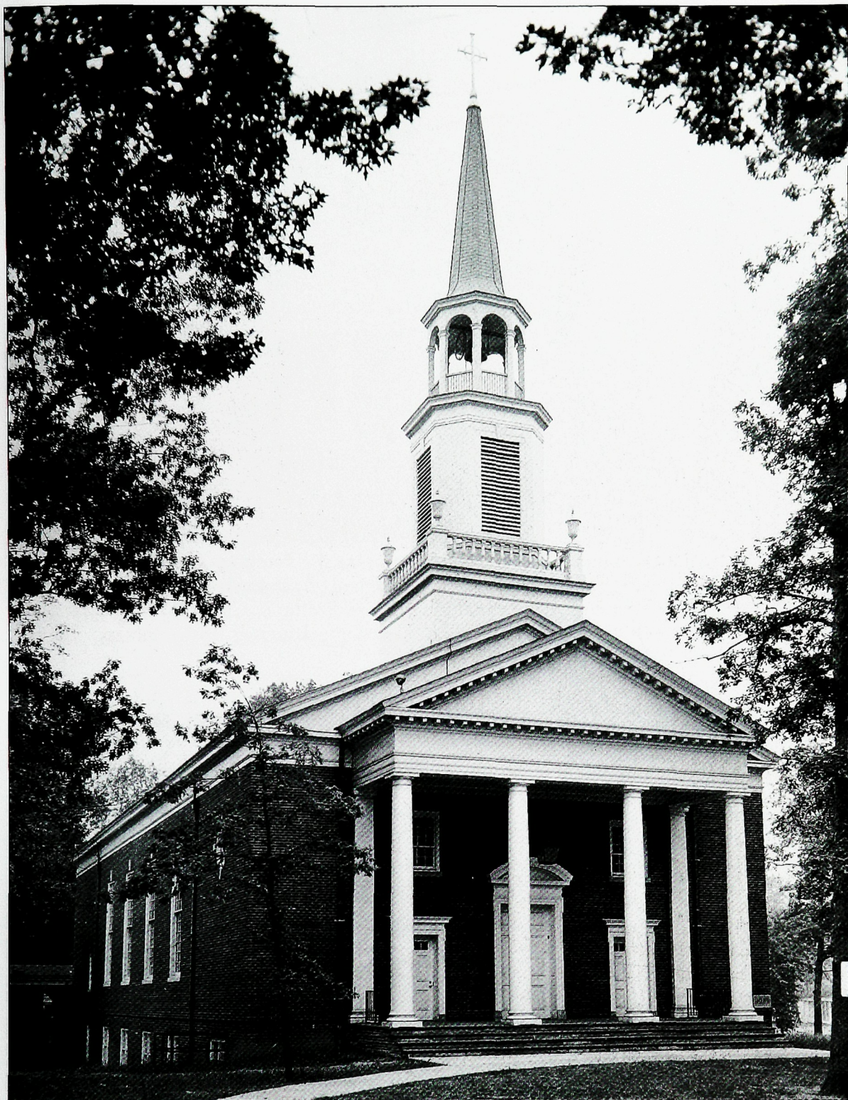
ITS STATELY SUCCESSOR. Mirroring the booming growth of the community during the post-war era, the Fanwood Presbyterian Church's congregation hailed from many states and many different religious affiliations. Outgrowing its original home, the sanctuary building of today was dedicated on September 21, 1958, with its front doors facing Martine Avenue.
