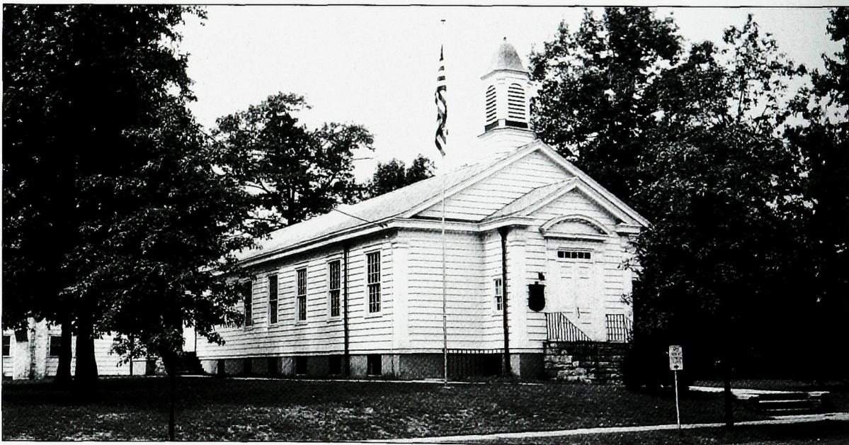
A LITTLE WHITE CHURCH. Dedicated on November 18, 1934, the Fanwood Presbyterian Church, on Marian Avenue, became the first church within borough limits. With membership on the rise, the church was expanded by 30 feet, and an education building was constructed in 1948.
