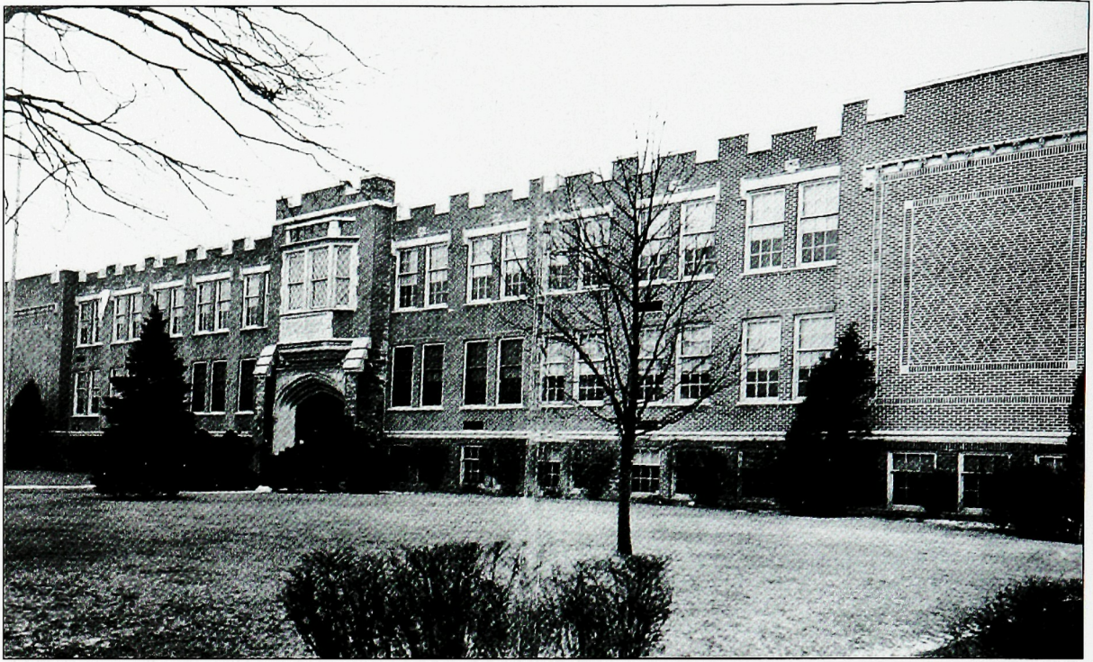
THE FIRST HIGH SCHOOL. Fanwood teenagers attended high school in Scotch Plains. This building was constructed in 1926 on Park Avenue and served as the high school until 1958. It became a junior high and is now a middle school for grades five through eight. Many alterations have been made to Park School over the years.
