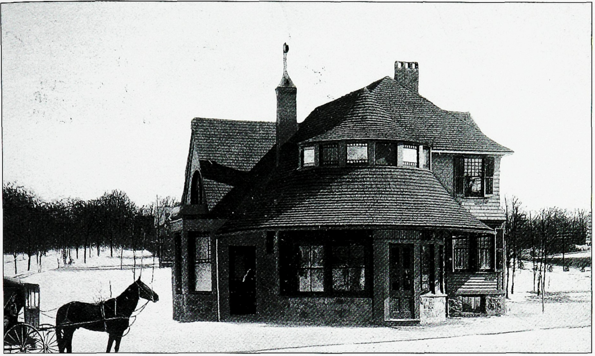
THE OLD POST OFFICE. The first Fanwood post office was built in 1897 in the Richardsonian Romanesque style. Located on Martine and North Avenues, this building is a traditional landmark of Fanwood. The rough-faced squared stonework, conical roof line, and large eyebrow dormer are its unique features. It was constructed by the Central Jersey Land Improvement Company and was given to the borough.
