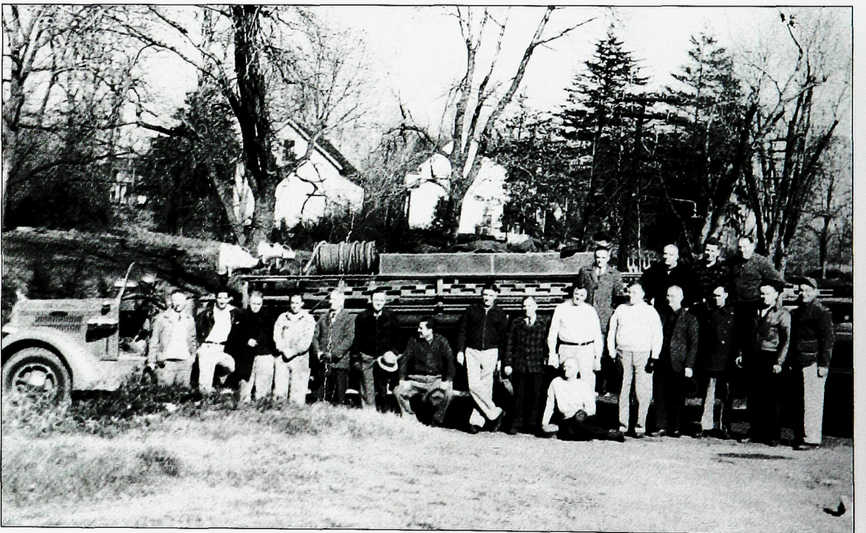
NEW EQUIPMENT. In 1936, the borough purchased Engine No. 2, which featured a fire pump, a water tank, ladders, and more than 1,000 feet of hose.
