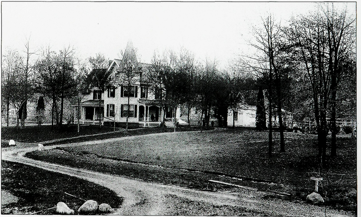
MAYOR YOUNG'S HOUSE. The residence of Fanwood's first mayor, Thomas Young, this house was located in the area bounded by Woodland Avenue, Forest Road, and Midway Avenue. It has since been replaced by contemporary homes.
