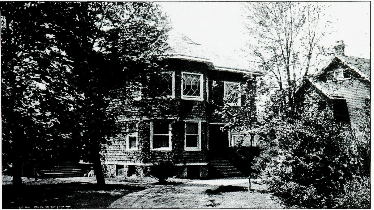
THE HOAR HOUSE. This Shingle-style house was home to W. H. Hoar, Fanwood's mayor from 1912 to 1917. Built in 1890, it bears several distinctive features. Eyebrow attic windows peek down on Fanwood's main thoroughfare, while the diamond-pane windows on the second floor give this Martine Avenue house a unique façade.
