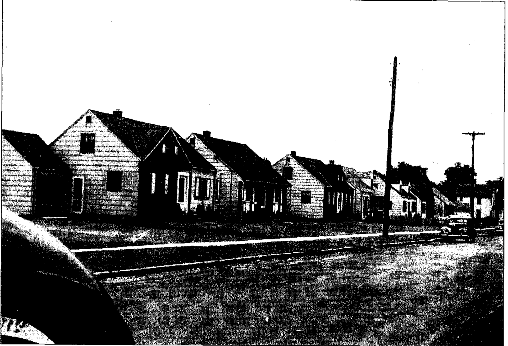
These newly-completed Cape Cod homes are of the standard bungalow design. They are still popular in Scotch Plains today.
