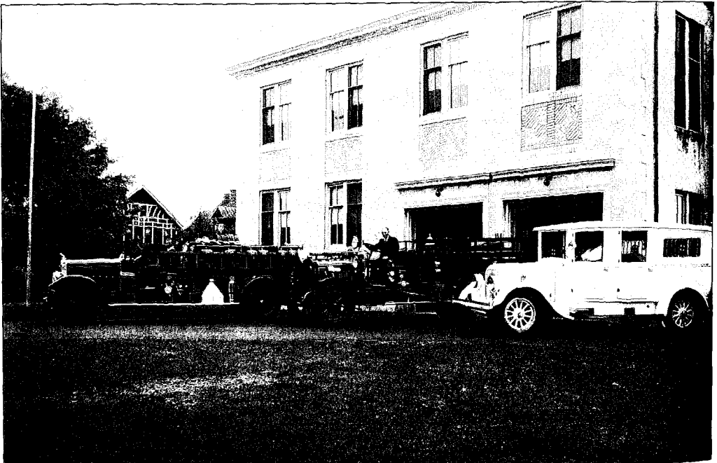
The Scotch Plains Municipal Building, c. 1930, showing fire and rescue equipment.
