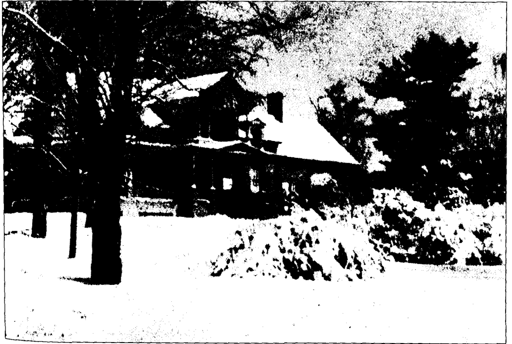
The J.H. Martine home during the winter, c. 1920. The piazza and dormers were added around 1900. The building was torn down in the 1930s.
