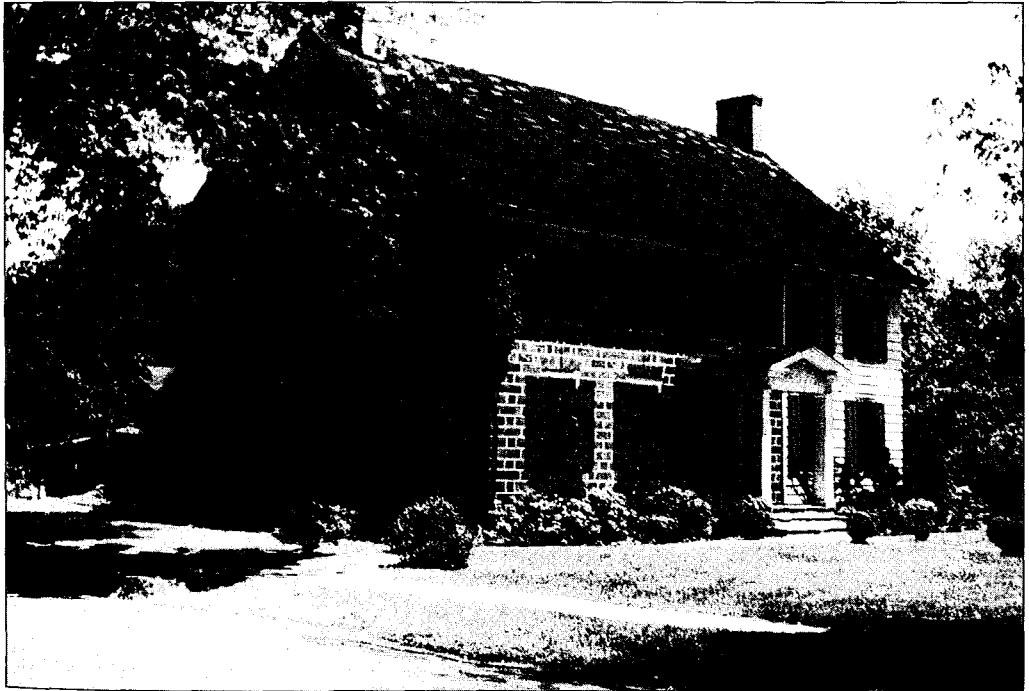
The Baptist Parsonage house showing the 1810 wood frame addition on the right side.
