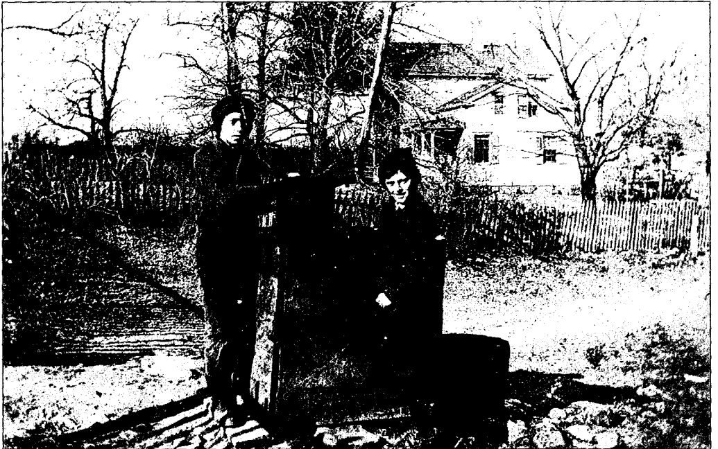
The Terry well (c. 1910). Another view of the well, showing the exterior wood structure, with two boys quenching their thirst. According to a member of the Terry family who still resides in Scotch Plains, the two boys are thought to be Elmer L. Terry (father of Peter Terry) and his brother, Herbert L. Terry, who died in World War I.
