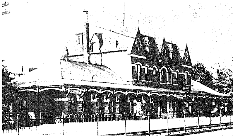
The Central Railroad Station enabled a large number of wealthy commuters and businessmen to make Plainfield their home.
