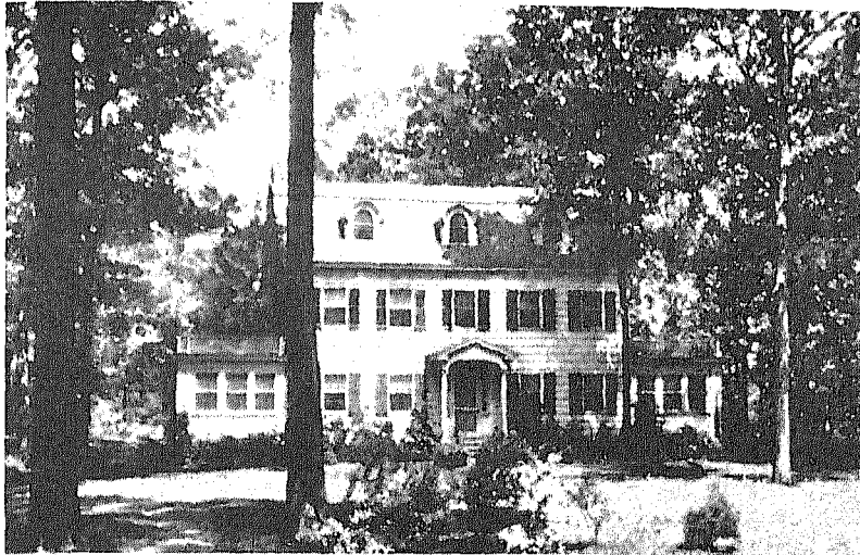
French style dormers set into a gambrel roof could be seen on the Thomas Preston residence on North Avenue.
