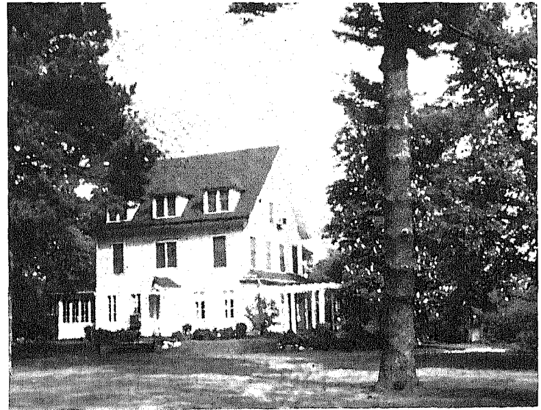
The Homestead was purchased from the Boucher estate in 1931 and was extensively remodeled for residential living by Mr. and Mrs. Clarence Slocum who eventually sold the property to the Borough in 1974.
