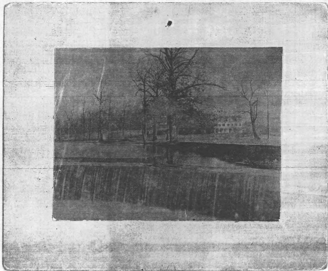
Marshes' Pond and the Marsh-Henderson-Di Donati House 175 Union Avenue (behind MacDonald's)
