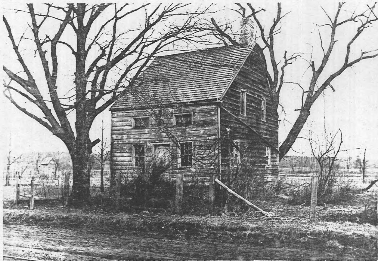
Old Marsh House, which stood on Westfield Avenue until 1942 when it was dismantled. Built about 1760. Picture taken in 1905. Scotch Plains, N.J.
